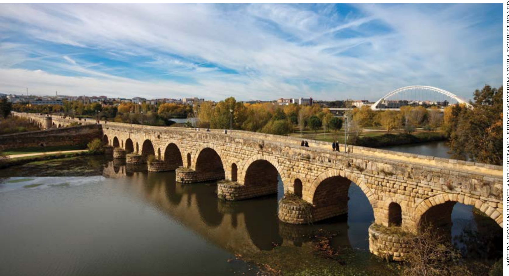
MÉRIDA (ROMAN BRIDGE AND LUSITANIA BRIDGE) ©EXTREMADURA TOURIST BOARD
